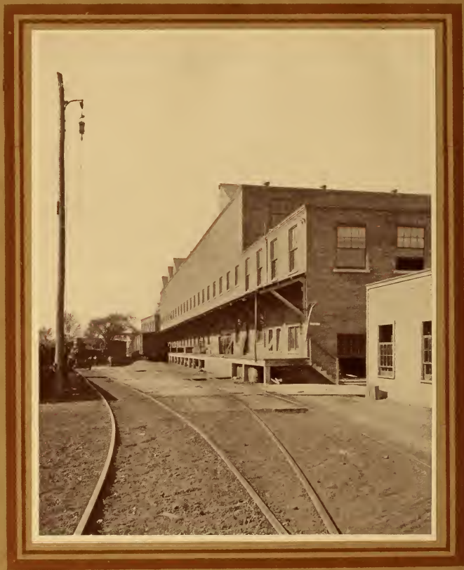
THE railroad warehouse, on a spur from the New York Central, is large enough for a town of several thousand inhabitants. This is used mostly for incoming freight, the outgoing goods being shipped from the State Street buildings, except glass plates in car-load lots which are shipped directly from the Park.
